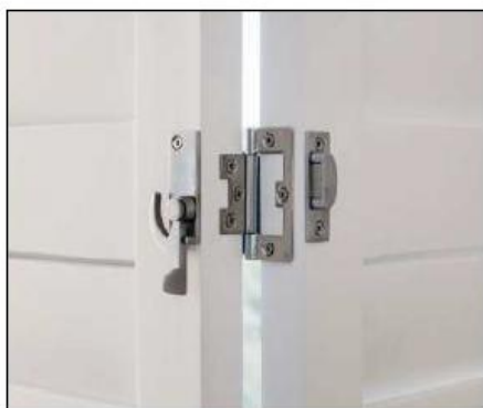
Hinges used to join shutter panels
